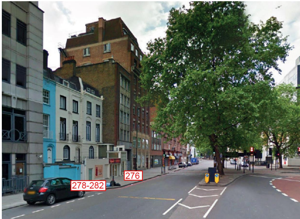
Facing south on Vauxhall Bridge Road
