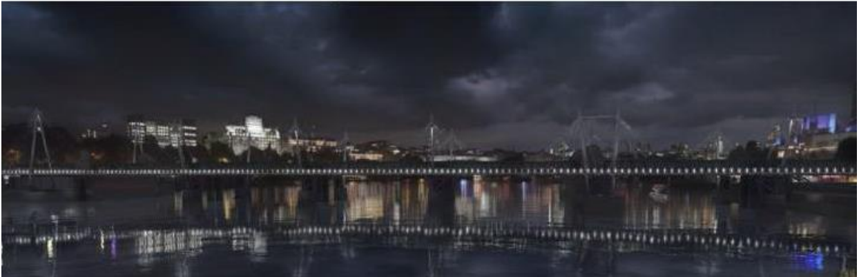
Golden Jubilee Bridge Illumination
